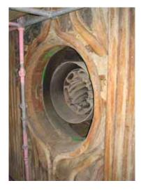
Photo 3. One of the 16 burners inside one of the furnace where boiler residues (white patches around the opening) were collected
